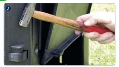
Press the connecting wedges into the snap-in hooks (possibly with the aid of a hammer).
